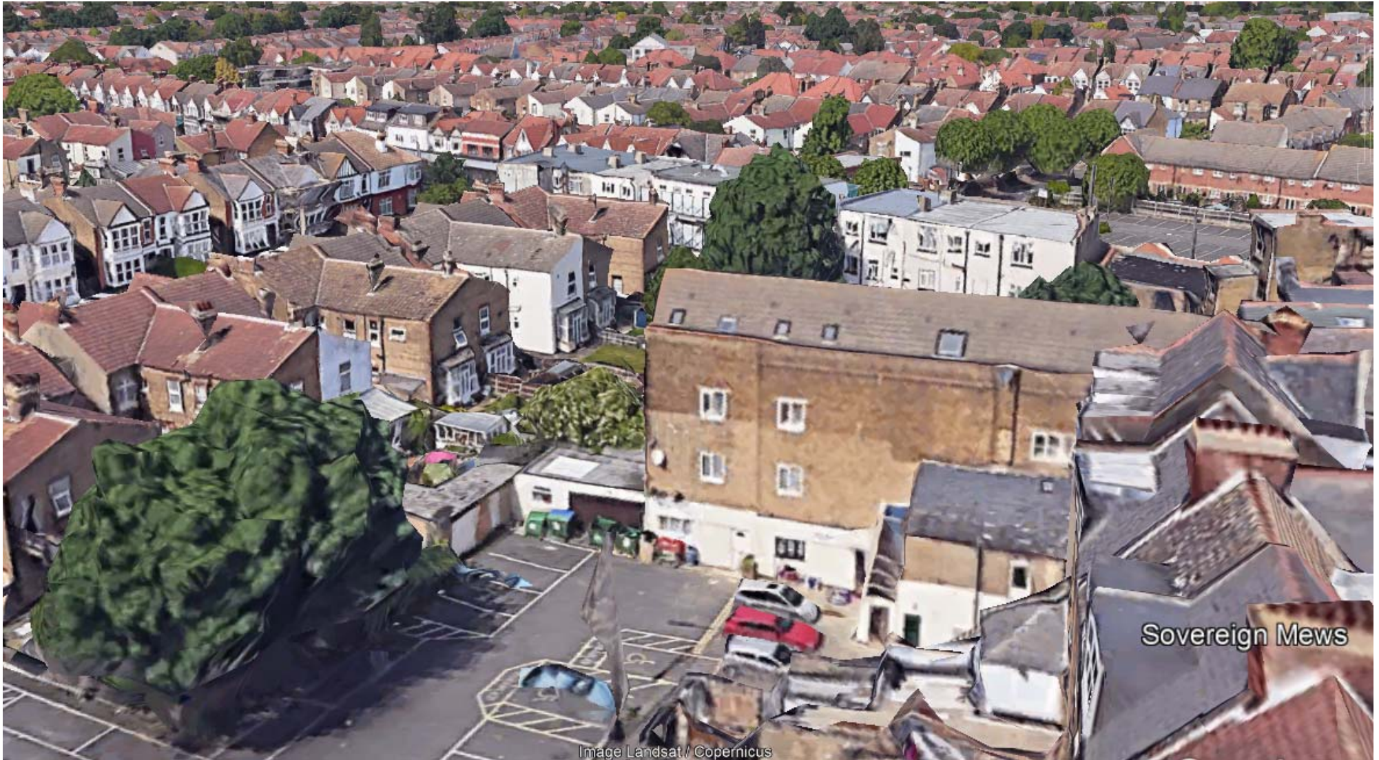
Rear of Sovereign Mews showing unauthorised flats to ground floor and potential overlooking from an unauthorised balcony to 1 st floor west elevation
